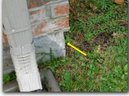
Wood was observed against the foundation wall. This is a condition that is conducive to attracting wood destroying insects. All wood against the foundation should be removed if practicable without damaging surrounding concrete; north side.
