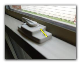
Observed one or more windows with deteriorating or missing caulk.
