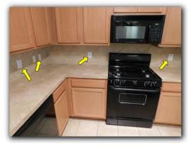
The Ground Fault Circuit Interrupter reset locations are; in garage for all garage and exterior outlets, in kitchen for kitchen counter top outlets and in master bathroom for all bathroom outlets.
